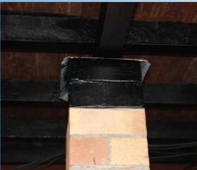
Creo-Fen Ten as a pier, bearer and Joist termite barrier to existing subfloors
